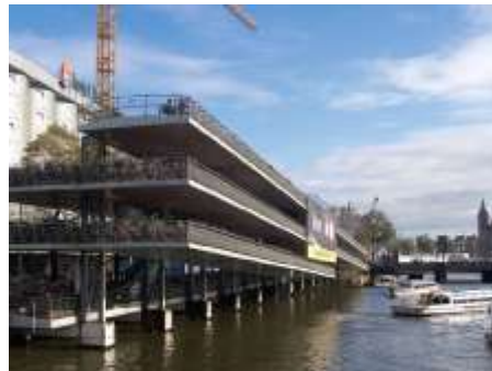
Amsterdam's innovative bicycle flat near the central station, built over water (NL)
