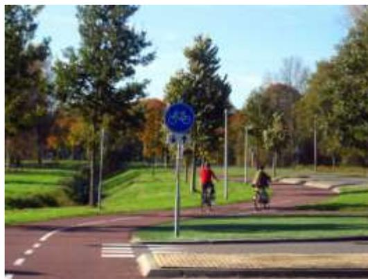
*Cycle crossing with a bent-out track (image source: P. Kroeze)*
