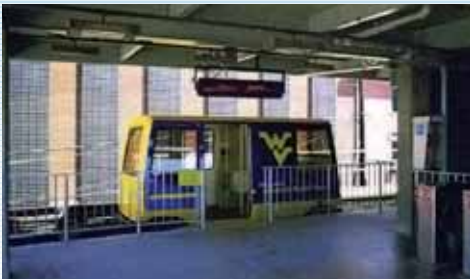
Morgantown GRT: an existing scheme serving the University of West Virginia, USA
