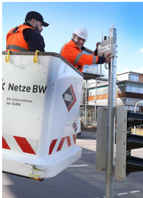
Figure 47: Road Side Unit (City of Stuttgart, Thomas Hörner)
