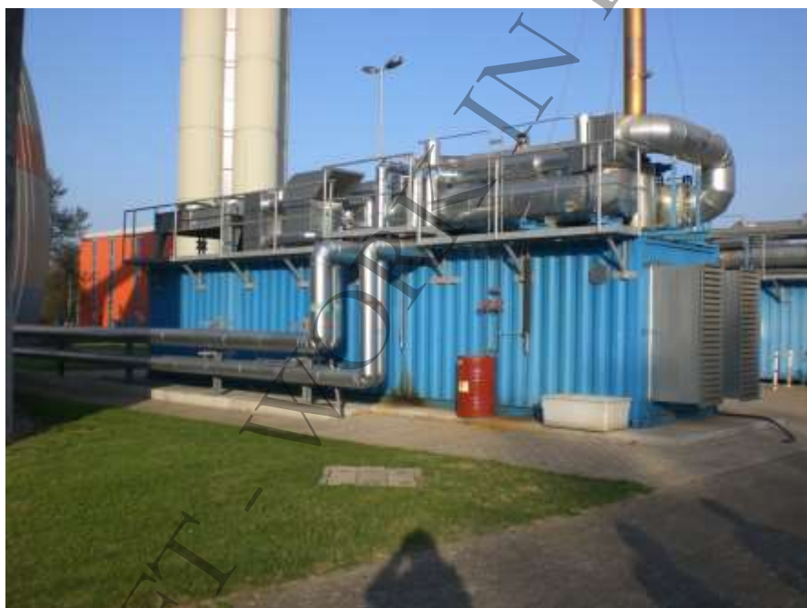
Figure 11-21: Retrofitted gas motor in a container for the use of biogas from anaerobic digestion of sludge to generate electricity and heat at the treatment plant “BreisgauerBucht”
