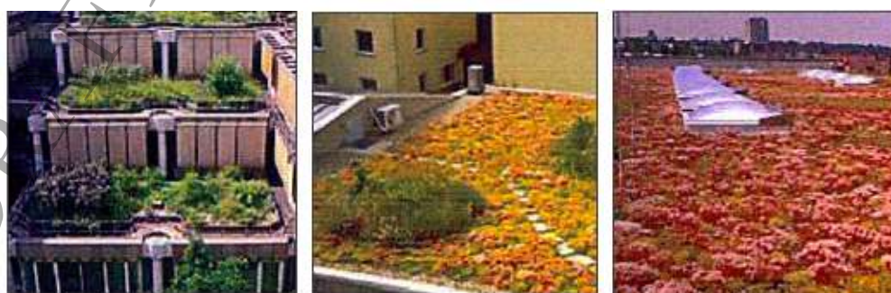
Figure 6-7: Types of green roofs; the order from the left is intensive, semi-extensive, extensive
