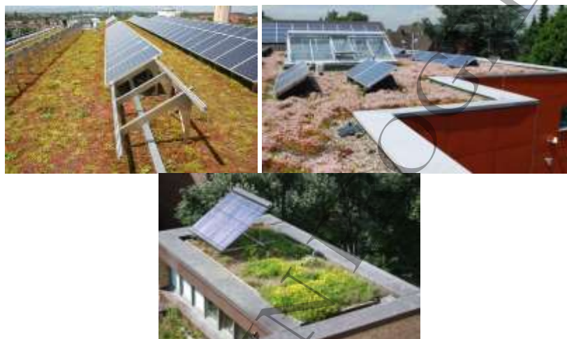
Figure 6-9: Combination of green roofs and PV panels; on the right picture a solar thermal panel is presented
