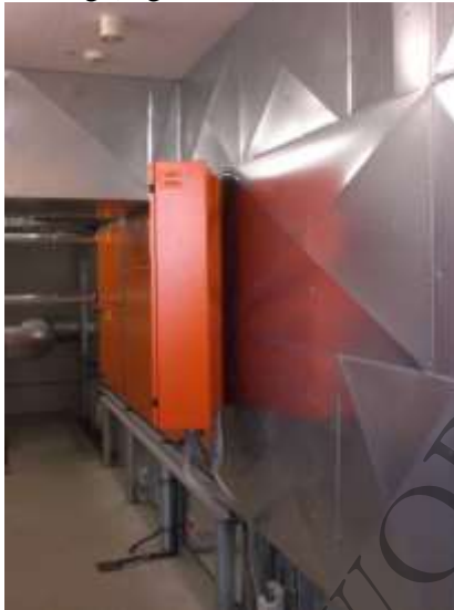
Figure 3-27: Exhaust air heat exchangers at Ridelberg school
