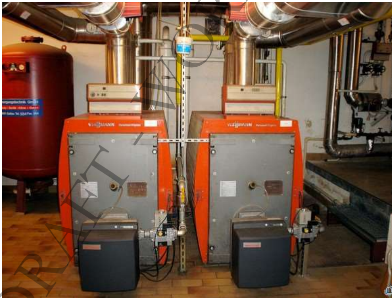
Figure 3-21: Gas boiler providing heating before renovation of Olbersdorf school (EnOB, 2010)
