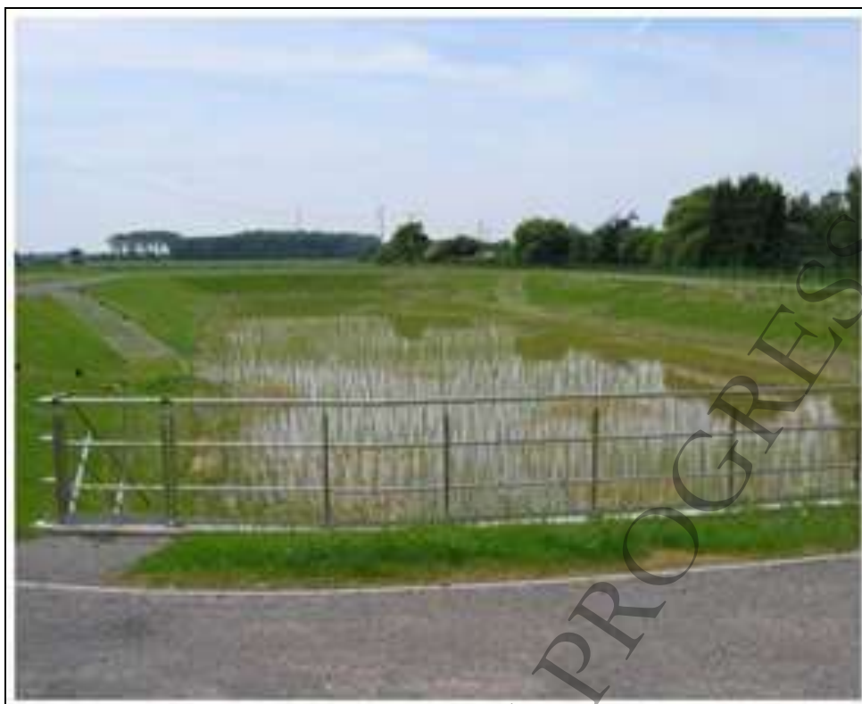
Figure 11-29: Retention basin (sedimentation) and retention soil filter for the disposal/treatment of storm water
