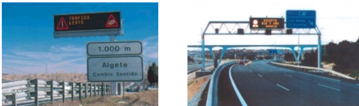
Figure 2: Real-time traffic information and management via VMS
