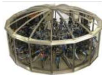
Bicycle mill in Nieuw-Vennep in The Netherlands: underground parking for 200 bicycles, in the form of a giant mill, 3m above ground, 9 m below. www.fietsmolen.nl
