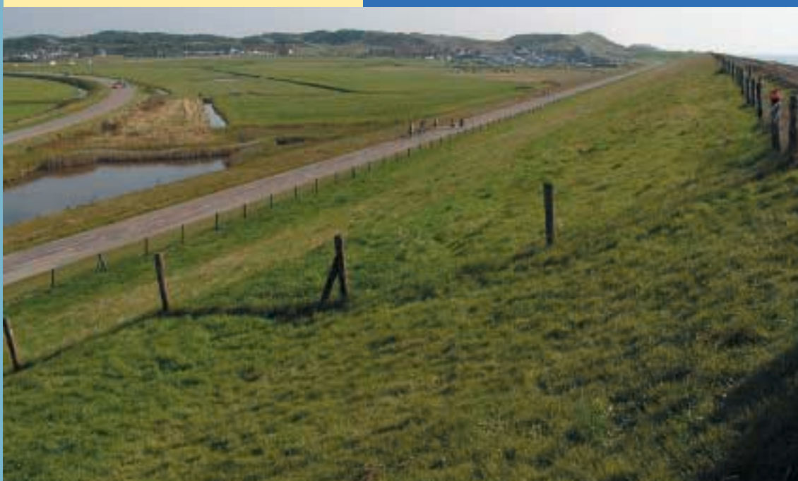
Hondsbossche Zeewering, one of the weak links.
